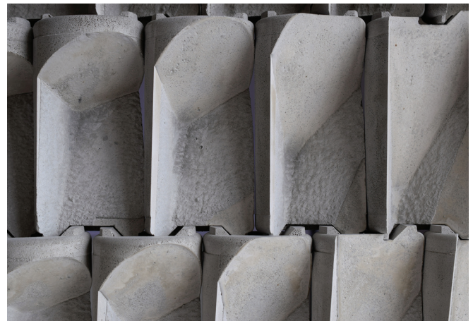
14 Detail view of prototype showing sections of open and closed bricks
