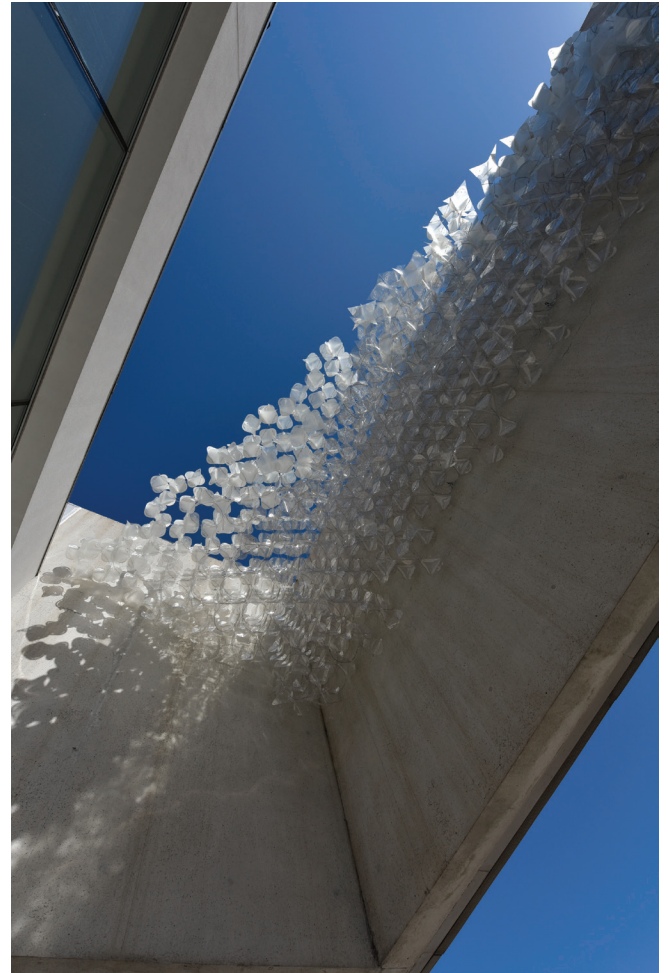
4 View into cantilevered corner.
