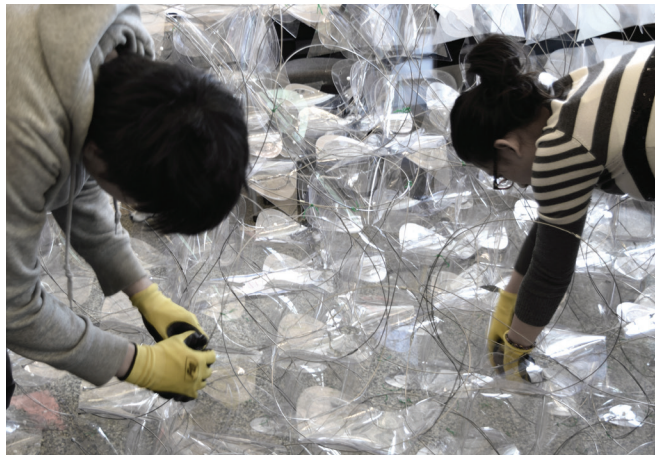
8 Snapping surfaces onto wire during assembly.
