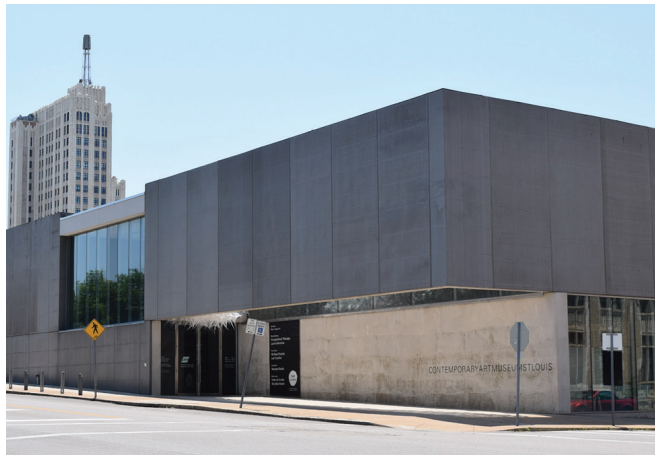
3 Site location inside cantilevered exterior void.
